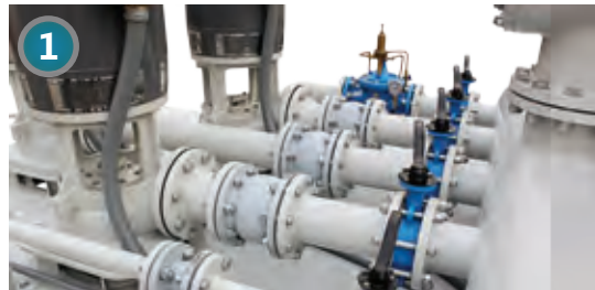
Silent wafer check Valves
